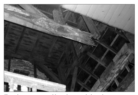
The northeast corner supports of the steeple were completely rotted away.
