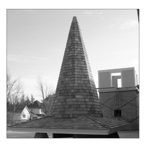
November  $16^{\text{th}}$ : With proper footings, new columns, replaced and reinforced beams, the new steeple was craned into place with only  $1\frac{1}{2}$  inches clearance between the church roof and edges of the steeple. With little wind, the start to finish of the crane's time installing the steeple was two and a half hours.
