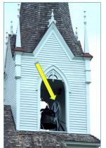
In May 2016, we replaced the old wooden wheel that rang the bell in the steeple of the 1894 church. It had rotted over 141 years, but that's not bad longevity, given that the wheel had a one year warranty! Thanks to skilled efforts by Himec Mechanical in Northfield, a replica of the original is now in place. They fabricated the white painted aluminum replacement wheel, and installed it with help from River City Builders.
